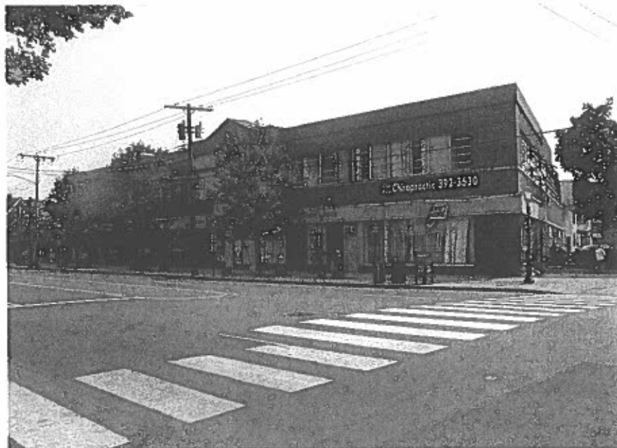
Extensive Fire Damage at 566 Whalley Avenue
