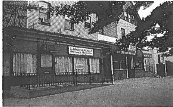
Substantial reinvestment made at 383-385 Whalley Avenue
